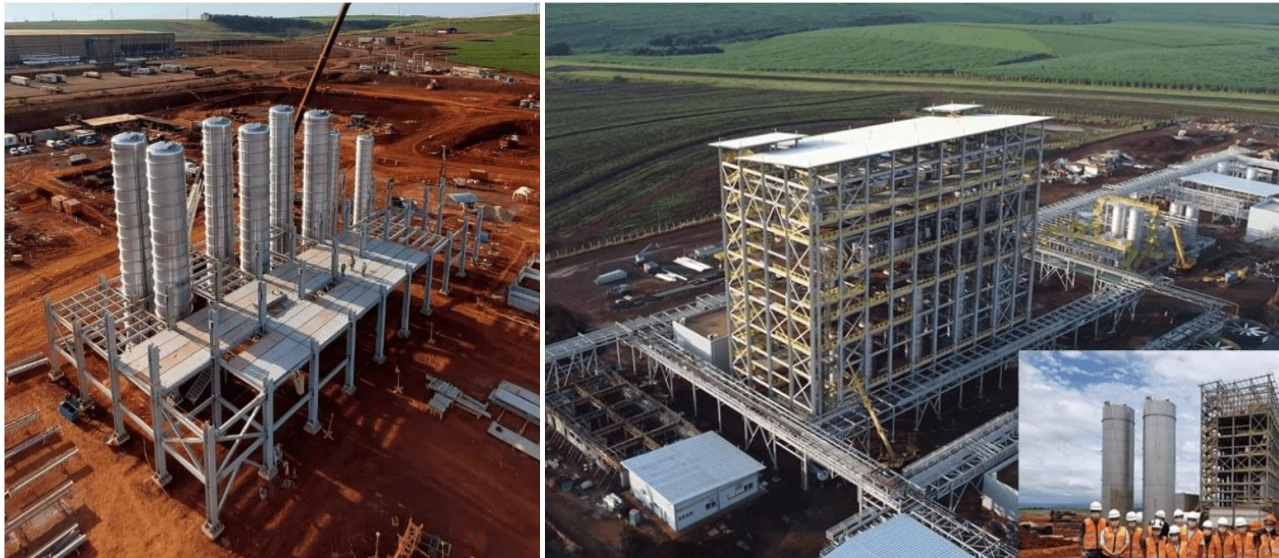
Barra Bonita Fermentation Facility
